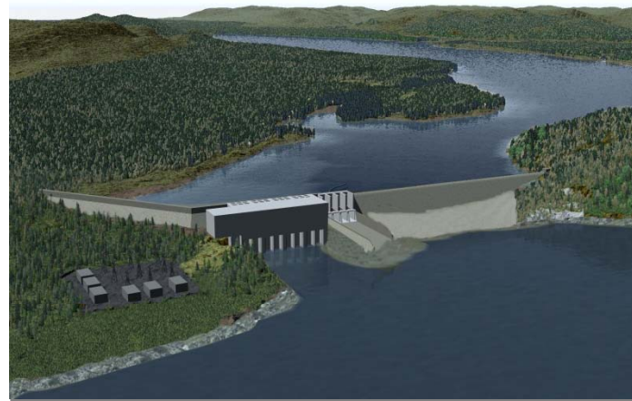
Two dams and powerhouse at Muskrat Falls
